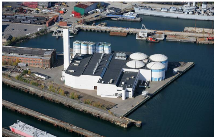
Figure 1: MWRA's Pelletizing Plant
