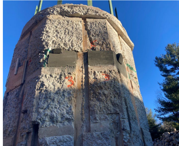
Repairs to the 1927 octagonal structure
